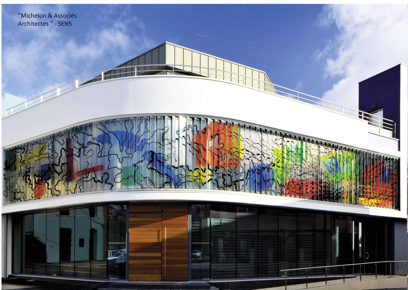
Architecte: Vial Gaivoronschi
